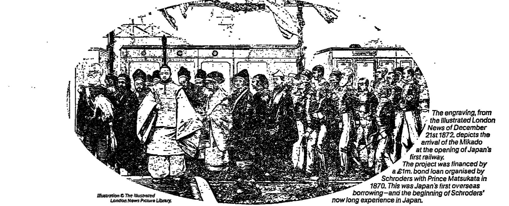
The engraving, from the Illustrated London News of December 21st 1872, depicts the arrival of the Mikado at the opening of Japan's first railway. The project was financed by a £1m. bond loan organised by Schroders with Prince Matsukata in 1870. This was Japan's first overseas borrowing—and the beginning of Schroders' now long experience in Japan.
